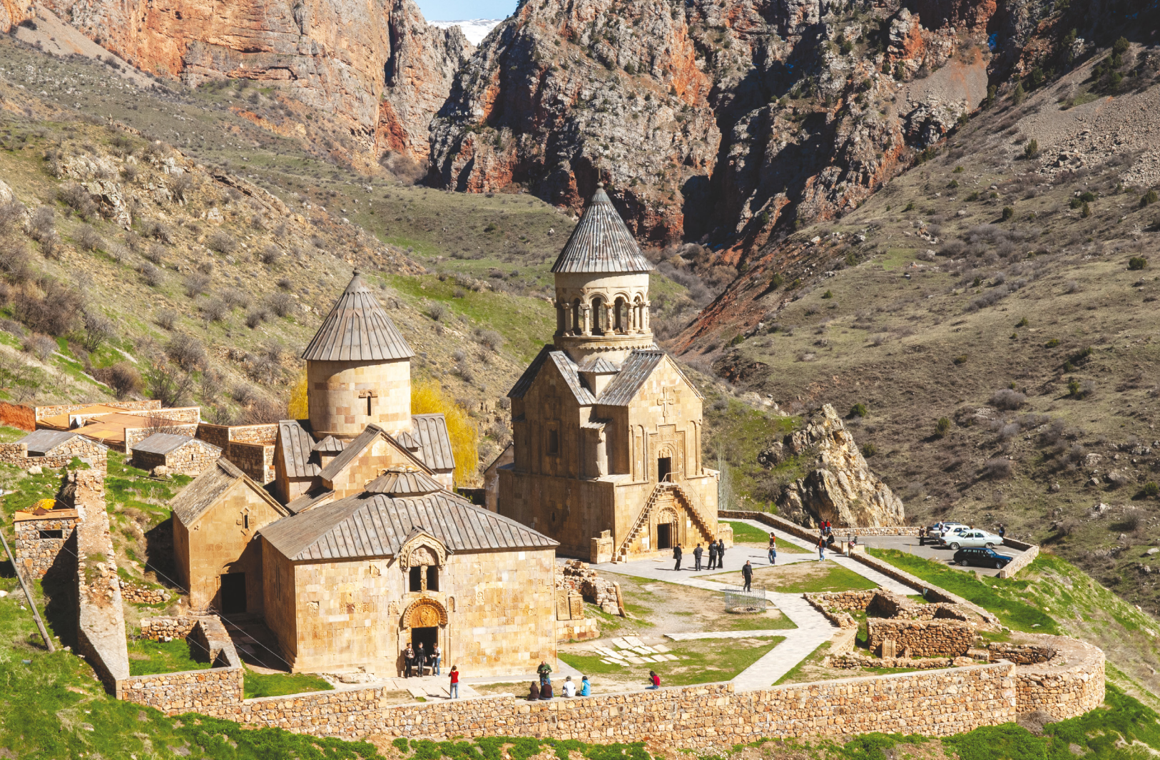
[fig. 3b] A view from above of the Noravank' Monastery, 12 th –14 th century
