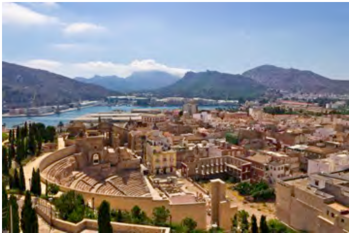
Figure 15a. Moneo, Plan and cross-section, Museum of Roman Art, Merida, Spain, 1980-85. Figure 15b. Aerial view of the Roman Theater.
