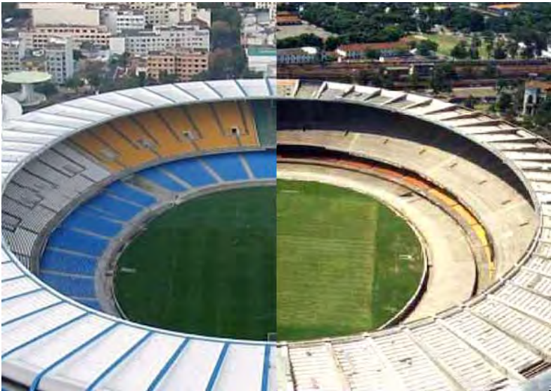
Figure 22. The stadium after and before the refurbishment of 1992.
