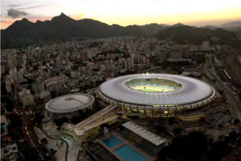
Figure 1. View of the Maracanã complex. Credit: Fernandos Arquitectos
