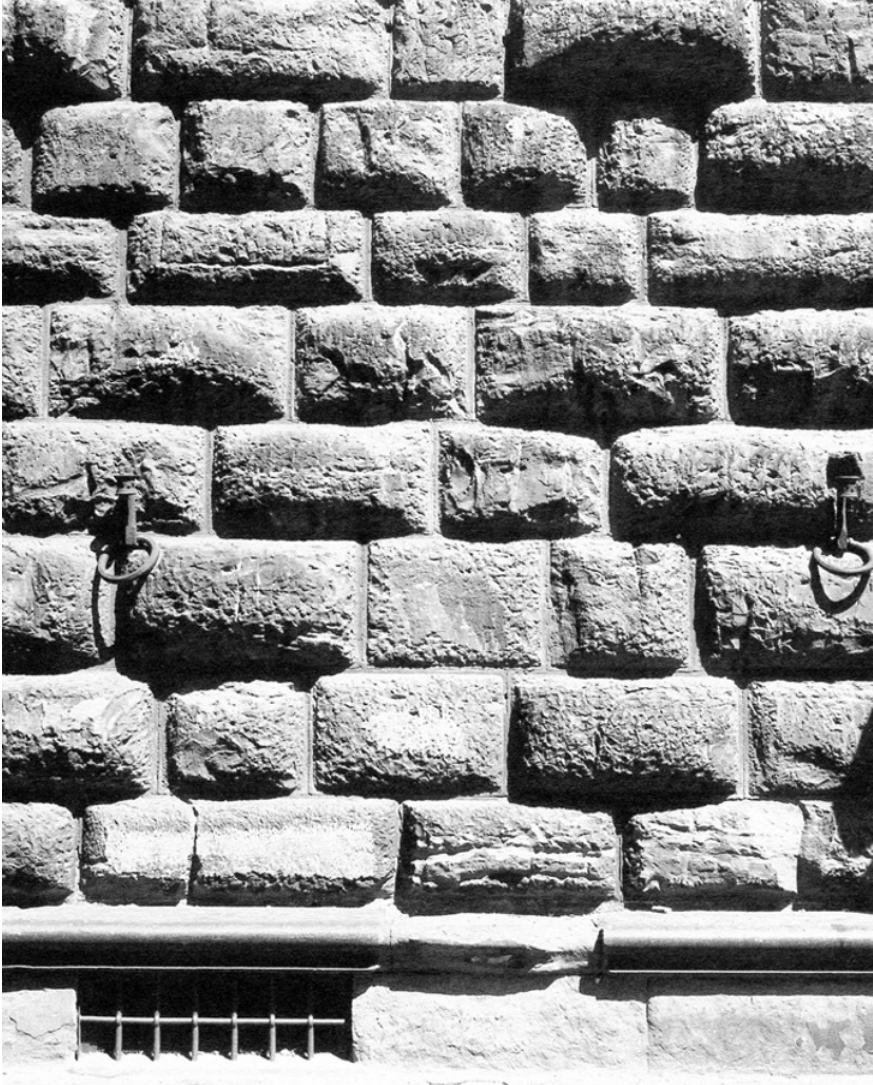
FIGURE 11.6 Medici Palace, the façade on via Larga. The bugnato of the ground floor.
