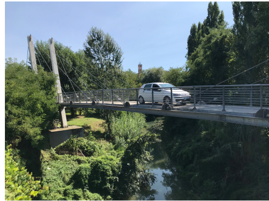
Fig. 14. Test of the bridge using a small car as load.
