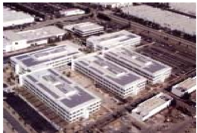
Fabbrica Toyota in California, Powerlight System
