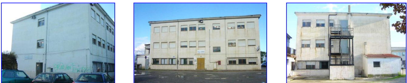
Fig. 1. Views of the building.
